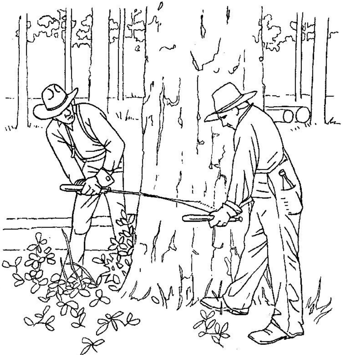
Men used **crosscut saws** to cut the large trees. Each crosscut saw required two men to **operate**. A man took a handle at each end of the saw and pulled back and forth until the tree fell. Notice the size of the trees. They were much larger than trees are today.
